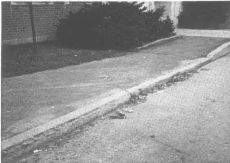
FIGURE 6: Comparative view of granite (to the left) and concrete (to the right) curbing.
