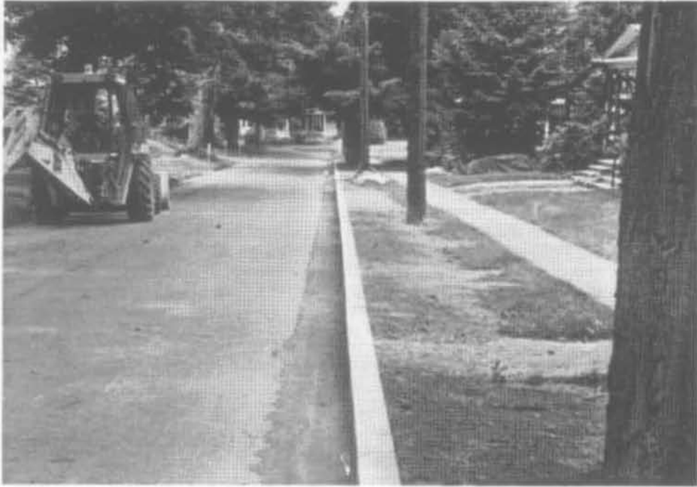
FIGURE 3: Modern machinery and methods produce granite curbs with neat sawn tops and smooth split faces adding to the aesthetic appearance of the pavement.
