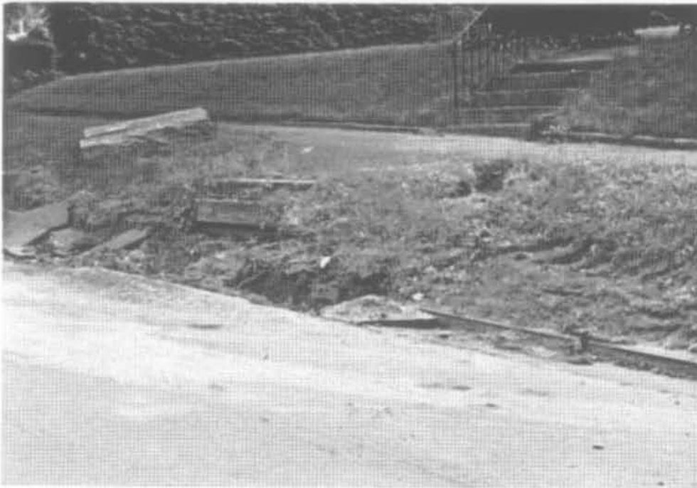
FIGURE 4: Due to its long life span granite curb can be removed and reset to new line or grade.
